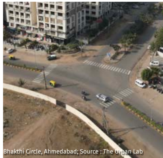
Three-leg Intersection (T-junction) Connects a minor road to a major road; simple layout with controlled turning movements.
